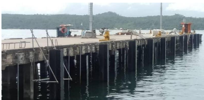
View of the Kudat Port Jetty
